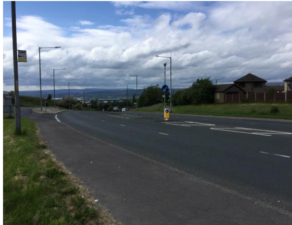
Rossendale Road with lay-by and bus stop adjacent to the site
