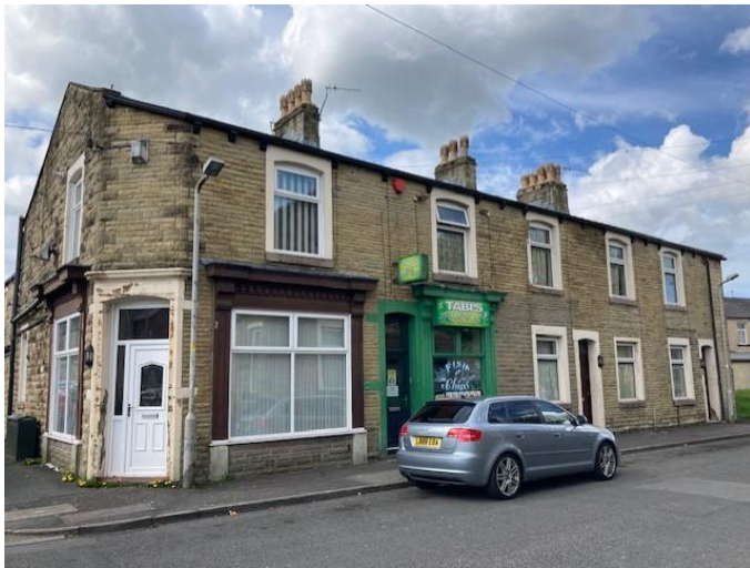
Photo 1: existing front elevation (April 2022)
